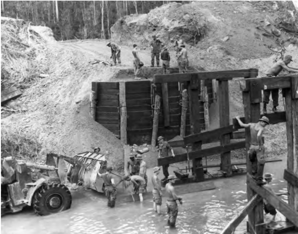
Bridge under construction along Route 547
